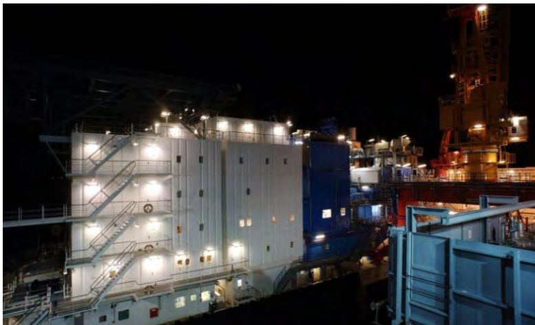
Figure 4: Living quarters prior to optimisation (Photograph: Studio B8 on behalf of RWE Dea AG).
