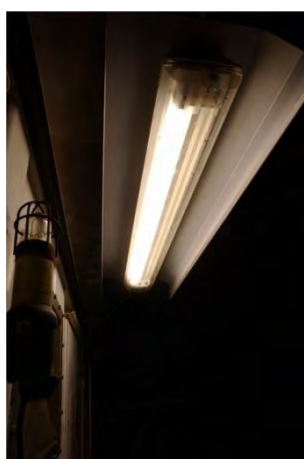
Figure 8: View of a lamp on a standby electricity generator with light guidance shield and illumination to half (Photograph: Studio B8 on behalf of RWE Dea AG).
